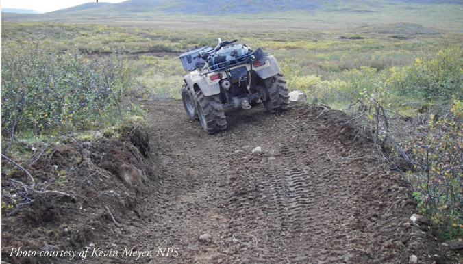
A super-elevated turn built into the tread of the Glacier Gap Trail.
